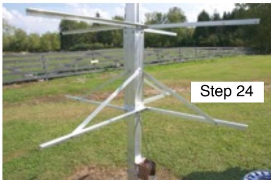
have a hole punched at each end (B). We will be attaching this angle so that the corner of the angle is facing the ground. Match the hole on the end of the angle (B) with the hole on one of the upper ring support about 7" in from the end. Insert a  $\frac{1}{4} - 20 \times \frac{3}{4}$  bolt add the nut. Place the opposite end
