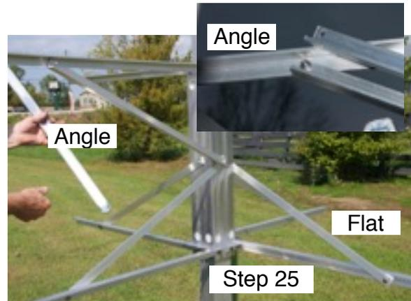
**Step 26)** Tighten all nuts and bolts that you have used to this point.
