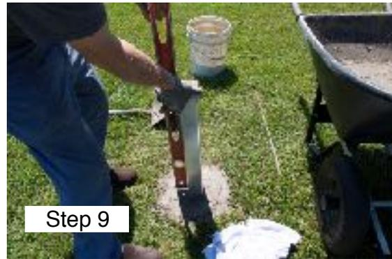
**TIP!** Before sliding your aluminum pole over the aluminum stake spray WD 40 or use engine oil on the aluminum stake.
