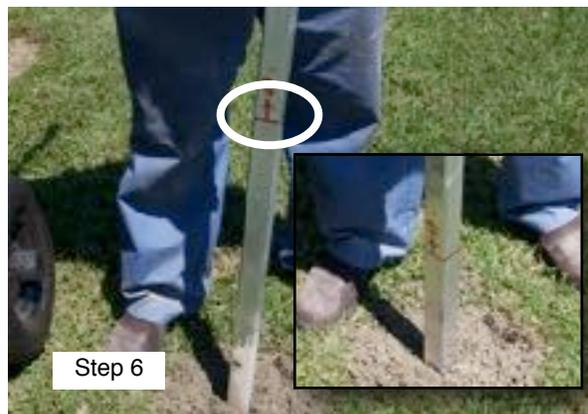
**Step 7** Wipe off any concrete from the exterior of the ground stake, check for level on 2 sides and that your ground stake is the full 24 inches above ground. Periodically check your ground stake for plumb. For best results wait at least 2 days for your concrete to cure.
