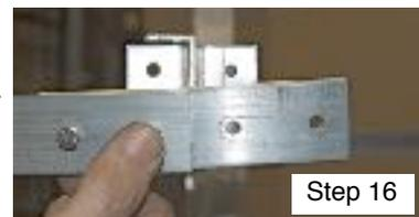
hole of the ring section, with the connecting bracket to the back side of the ring, place on a whiz nut. DO NOT TIGHTEN the bolts yet. You will want to repeat this process on both ends of the ring section you are working on as well as a second ring section.
