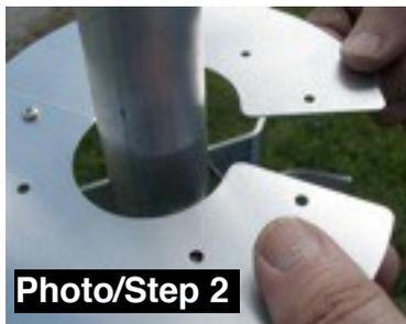
Step 2) Installing top plates using parts (A) top plates and 2 of the #8 x 3/8" (F) screws and 2 #8 nuts. Overlap the two halves so that the outermost holes align. Place one of your screws, through the top down and place a nut on and thread but don't tighten. Open the two halves and bring the top plates around the pole. (See Photo 2).
